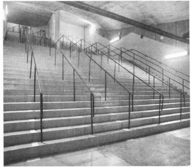
Main pedestrian entrance steps into the Mariaberget Civil Defence shelter in Stockholm
